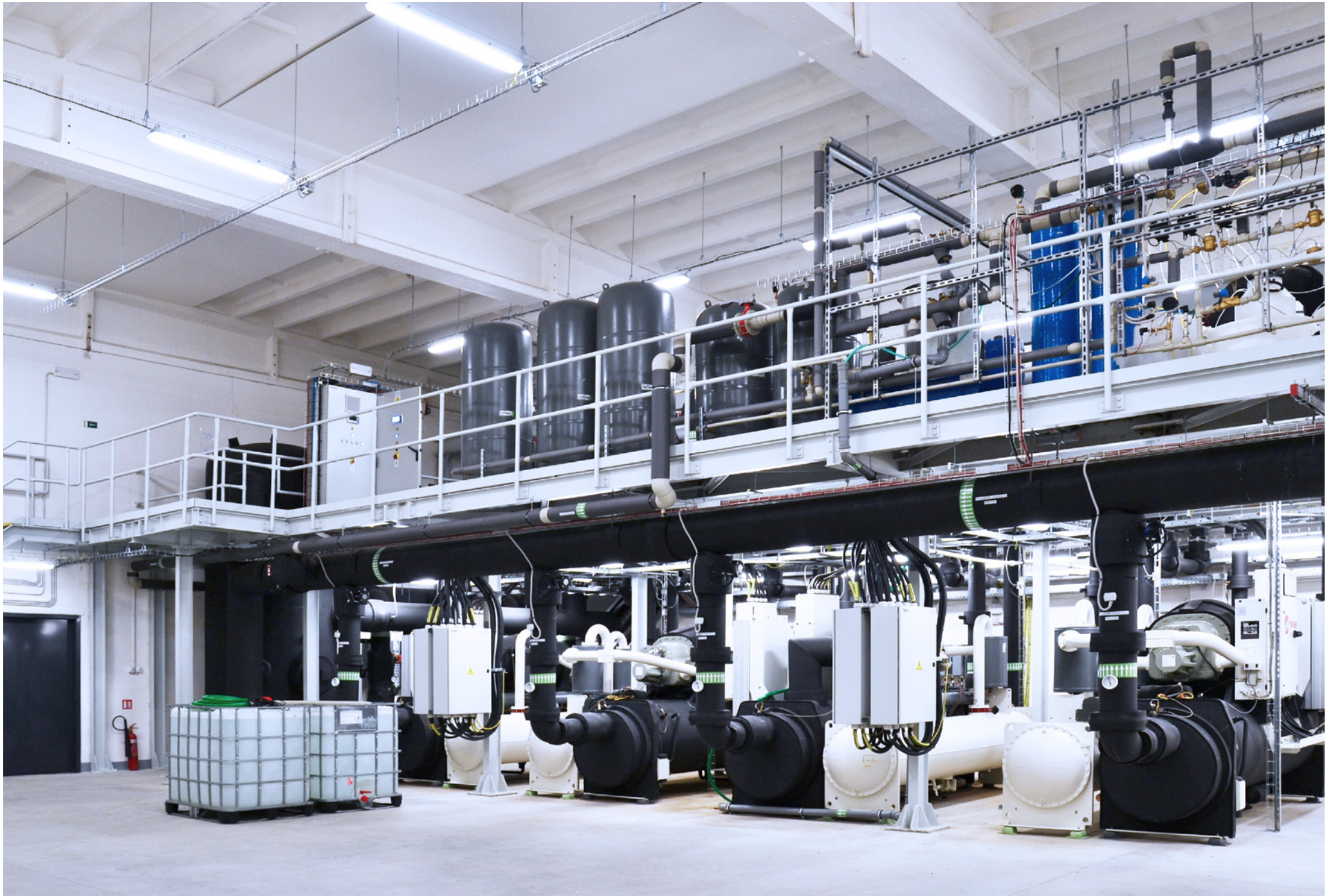
New source of cold for buildings M1, M8, M1 | ON Semiconductor Czech Republic, s.r.o. | Rožnov pod Radhoštěm, Czech Republic | 2018
