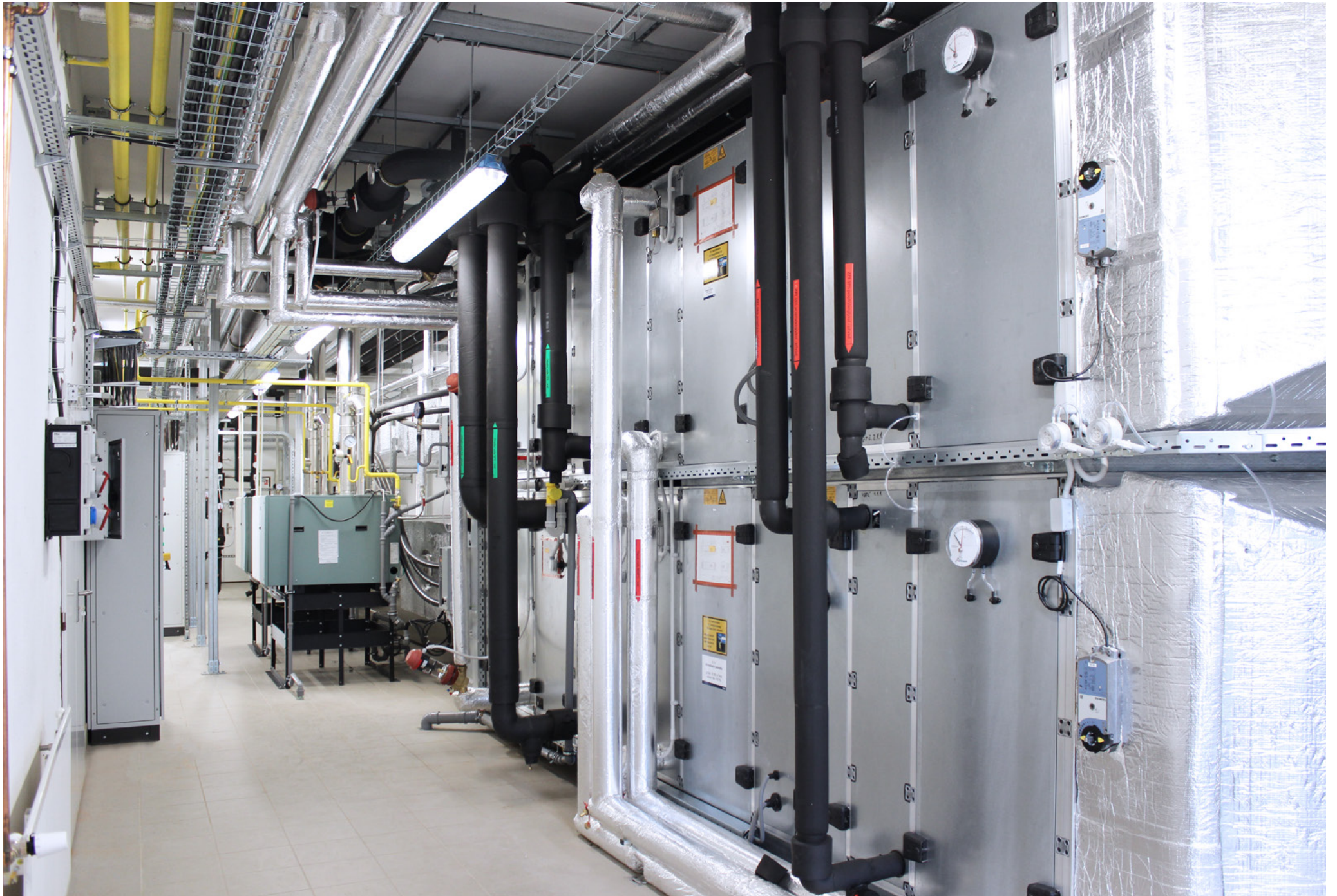
Production Building No. 163; Kayaku Safety Systems Europe a.s.; Jablůnka; Czech Republic; 2019
