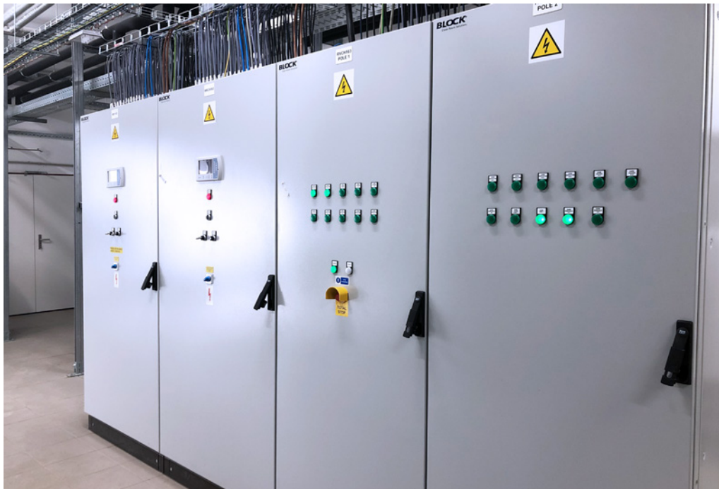
Production Bulding No. 163; Kayaku Safety Systems Europe a.s.; Jablůnka; Czech Republic; 2019
