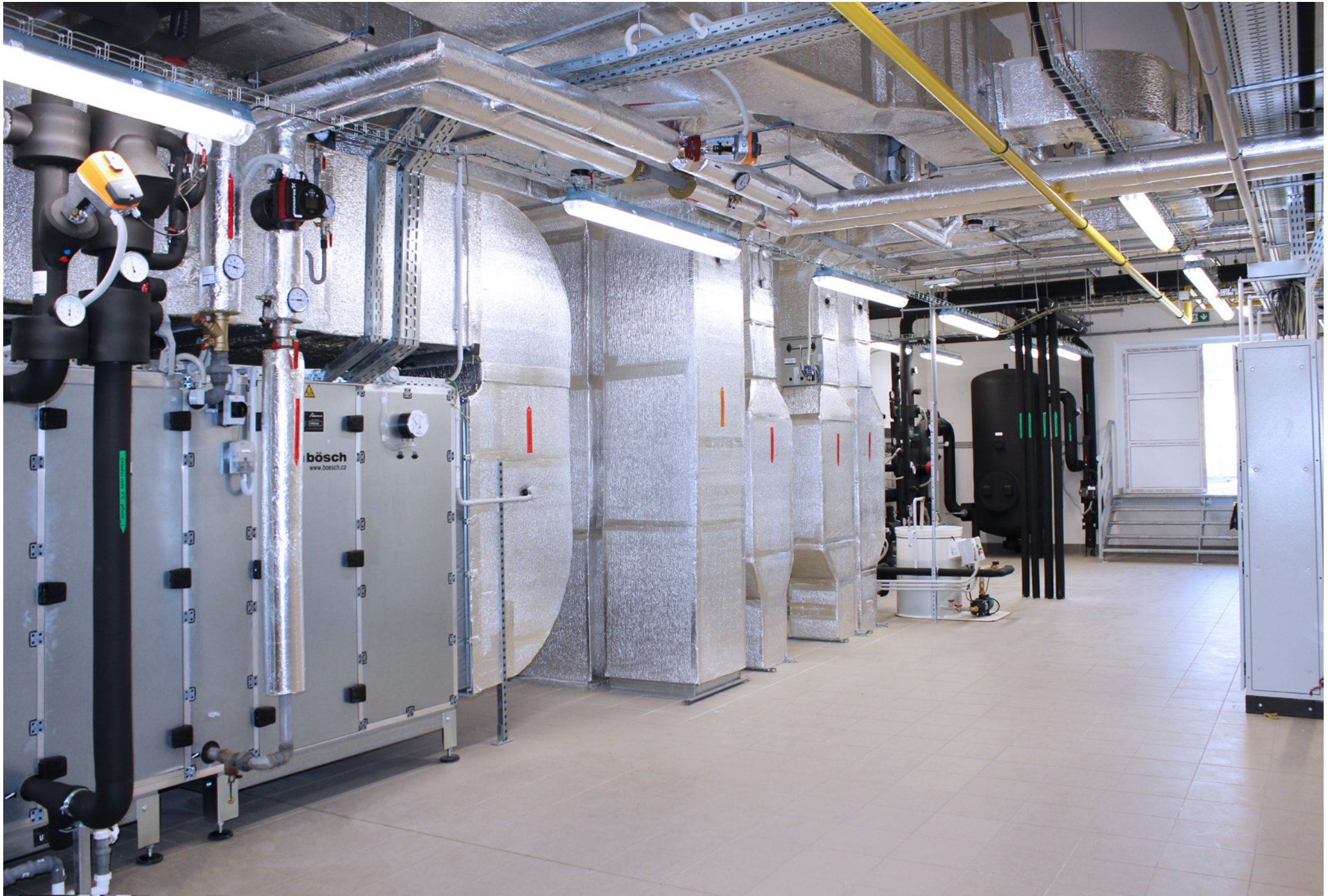
Production Building No. 105; Kayaku Safety Systems Europe a.s.; Jablůnka ; Czech Republic; 2019
